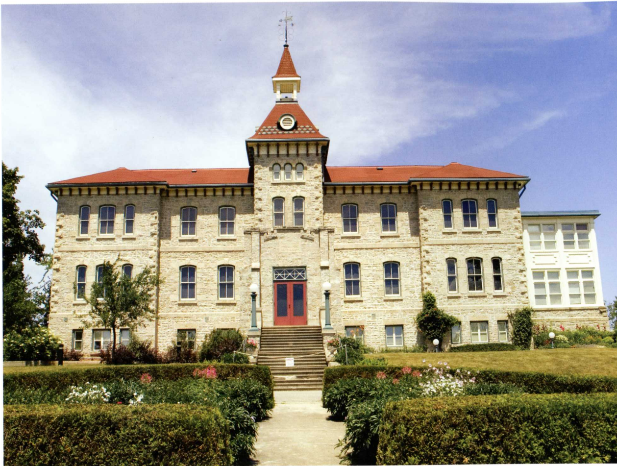
The 1877 House of Industry and Refuge, a National Historic Site, was designed by Guelph architect Victor Stewart in the Italianate Revival style. Noteworthy are its prominent belfry tower and rough-faced limestone construction. It now serves as the Wellington County Museum and Archives.
