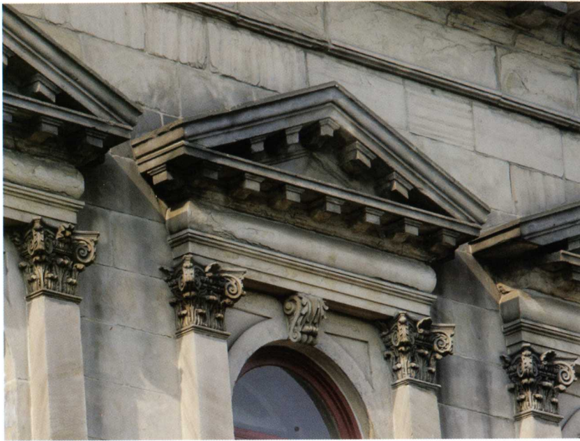
Both the Ohio sandstone, used on the Hamilton Custom House (left) and the local limestone used on the Guelph City Hall (right) can be more easily carved than most limestones.
