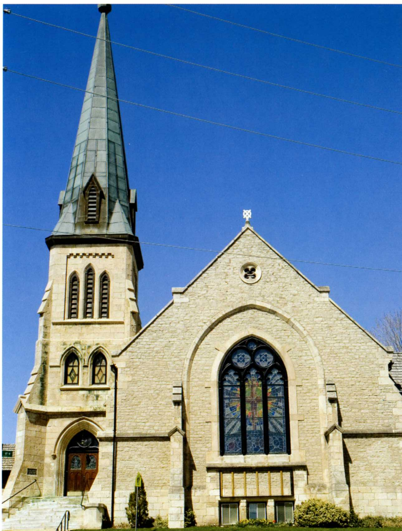
The 1862 St. Andrew's Presbyterian Church, designed by architect David Murray of Guelph, has a high nave and buttressed corner tower. The masonry combines the small, rough-faced Fergus stone with the lighter, smooth Guelph stone.
