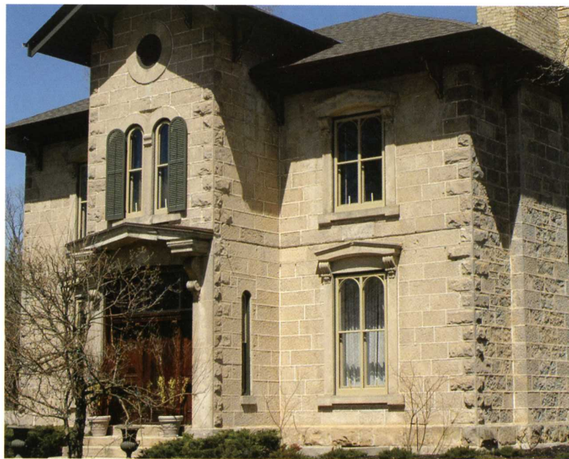
Squared limestone masonry is used in Inglebrook.
