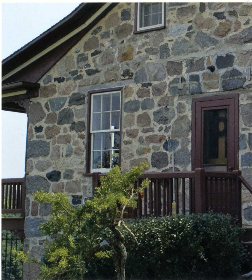
Fieldstone was the masonry preferred by the Mennonite settlers of Waterloo, as illustrated in this side view of the Swope House in West Montrose.
